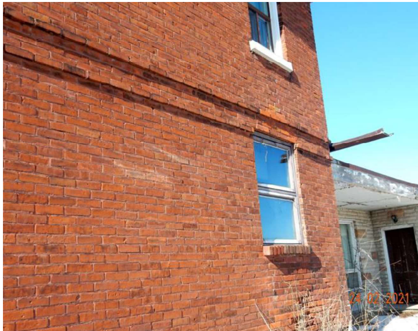
Figure 23: Detail, East Elevation, Double String Course & Later Window with Brick Arch and Sill, LDW
