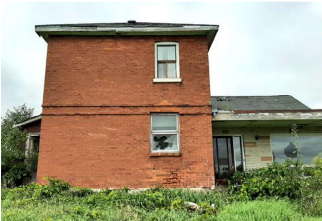
Figure 25: East Elevation, Rear Brick, Frame and Insulbrick Addition, Ground Floor Window (Later Insertion), Deteriorating Brick and Mortar, Town of Caledon Staff
