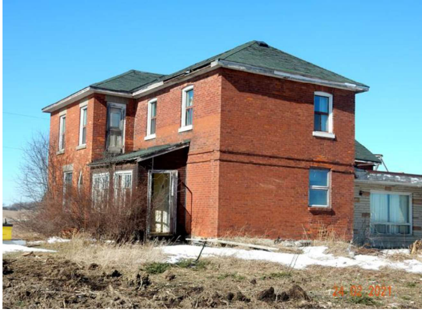
Figure 20: House, East Side Elevation Looking West with String Course & Entrance to Porch, Later Ell Addition to the Rear ,LDW
