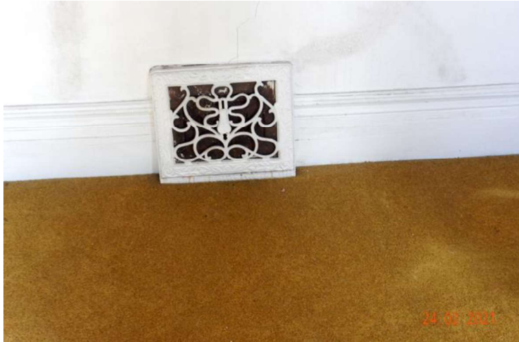
Figure 36: Old Iron Heating Vent & Original Baseboard, Main Floor, LDW
