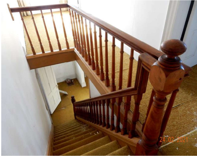
Figure 34: Staircase Railing and Newel Post, Modern Replacements, LDW
