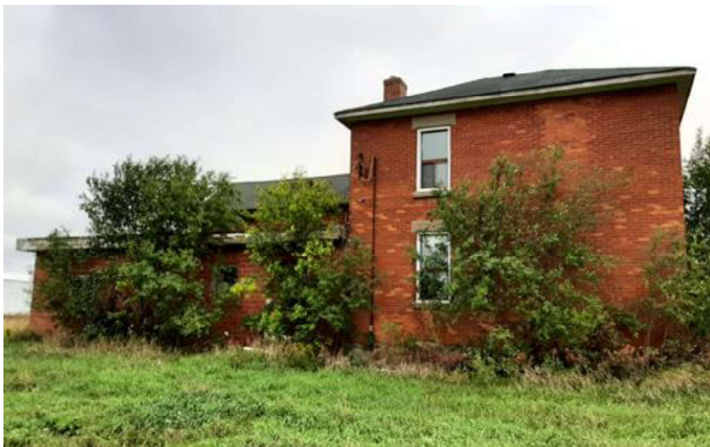
Figure 29: West Elevation, Bricked up Second Storey Window and Brick Rear Addition, Town of Caledon Staff
