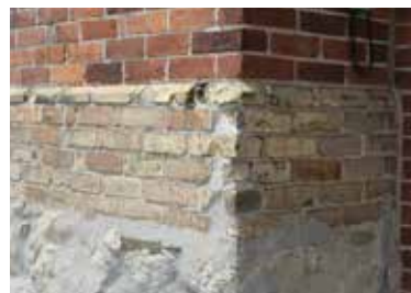
Brick deterioration on the east side of original portion of the building (ERA, 2018).
