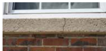
Cracked window sill on east wall (ERA, 2018).
