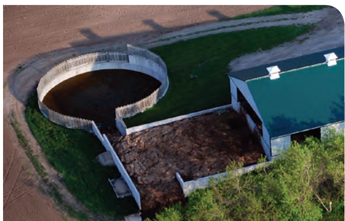
Figure 38. Uncovered liquid runoff storage (L1).
