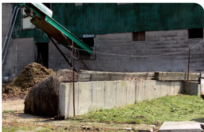
Figure 34. An uncovered solid manure storage with covered liquid runoff storage (V4).
