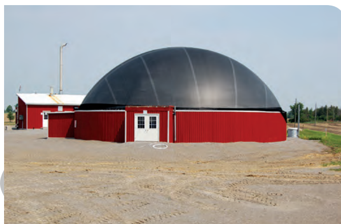
Figure 37. Raised base of liquid storage with tightly-sealed inflatable dome cover visible (V6).
