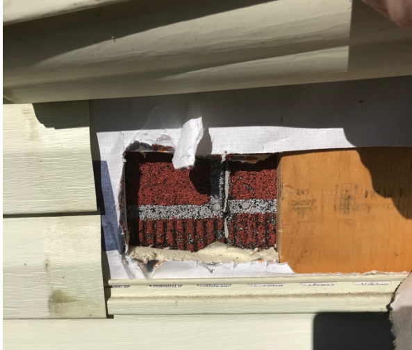
Figure 27a: Cladding below the vinyl siding is an asphalt and fibre product known as “Insulbrick”
