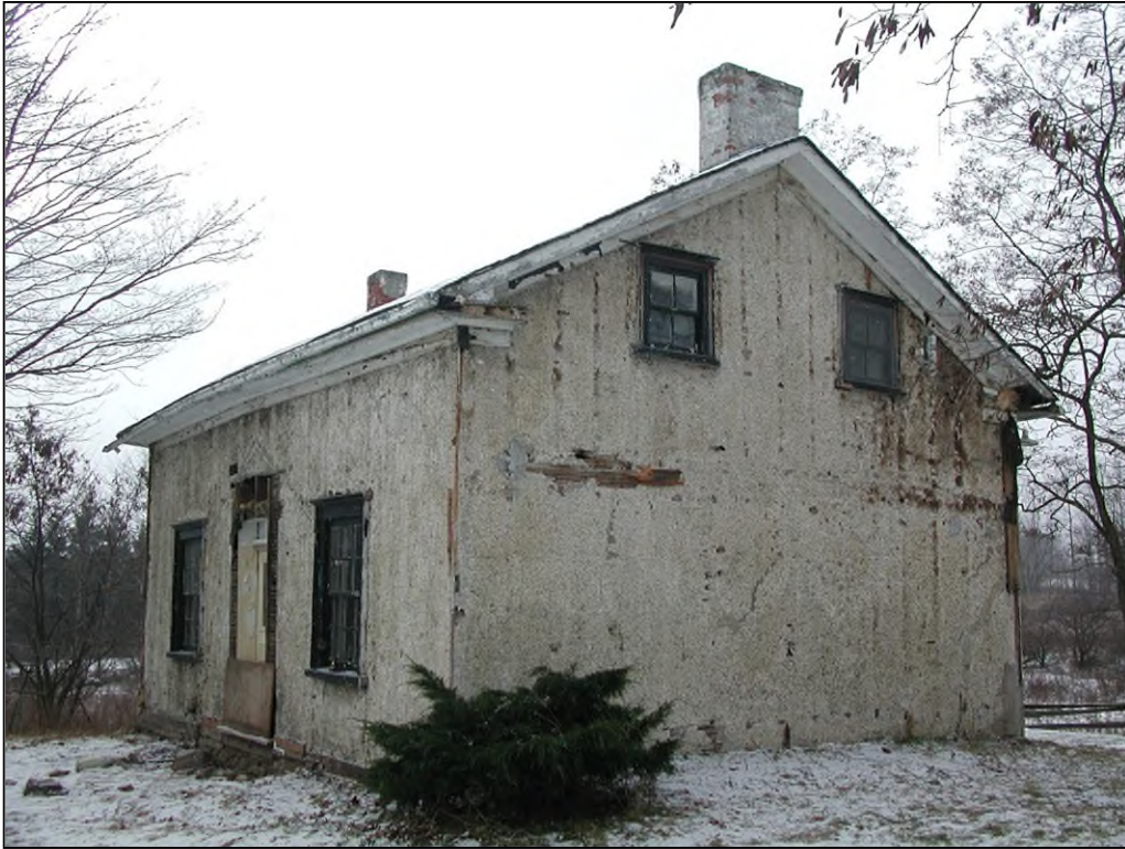
Figure 8: Above: East (front) and north facades showing original plaster cladding, December 2001 (Source: Andrew Stewart)
