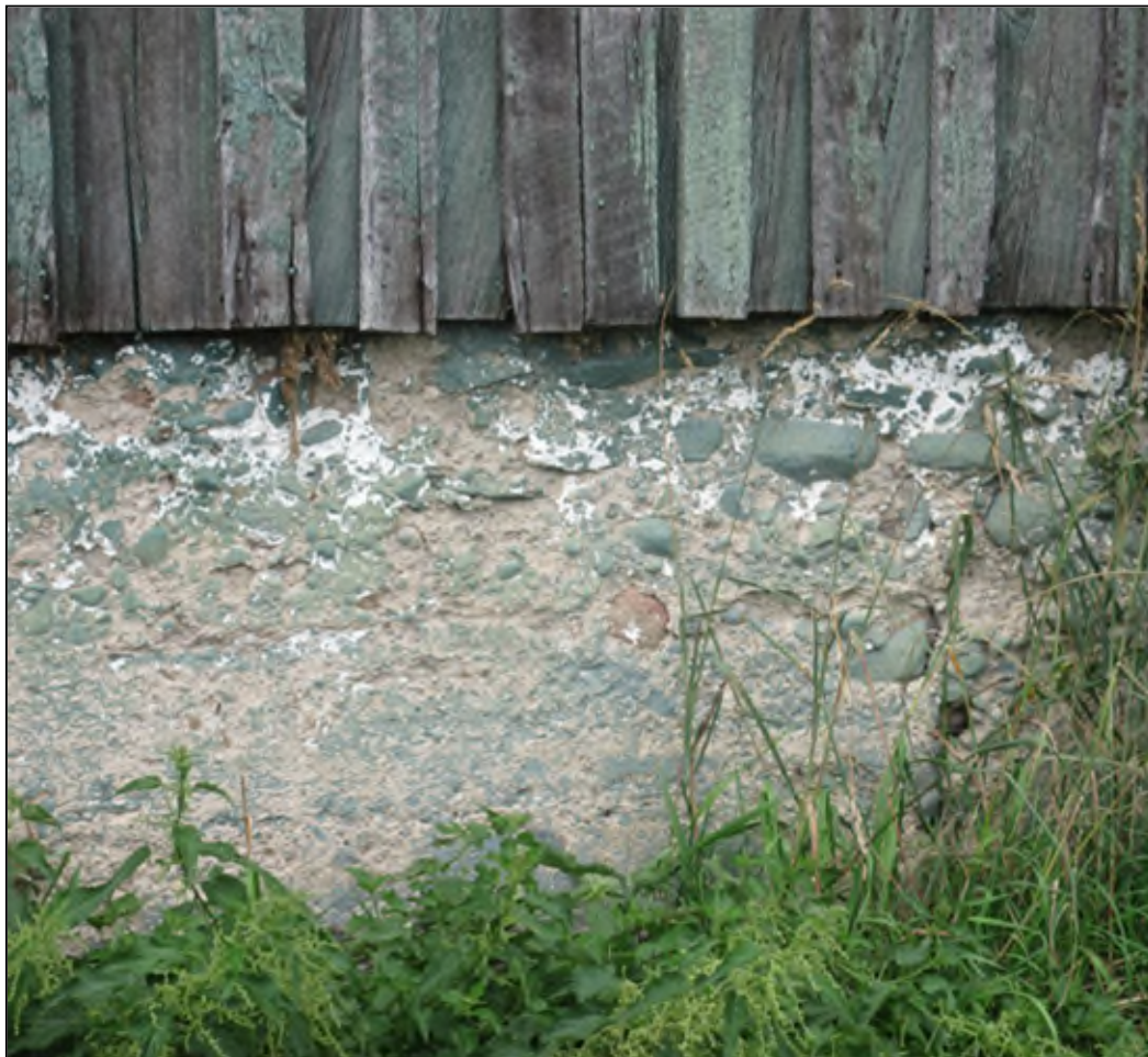
Figure 20: Section of foundation of main barn with rough stone aggregate concrete, July 15, 2021 (Source: Town of Caledon)
