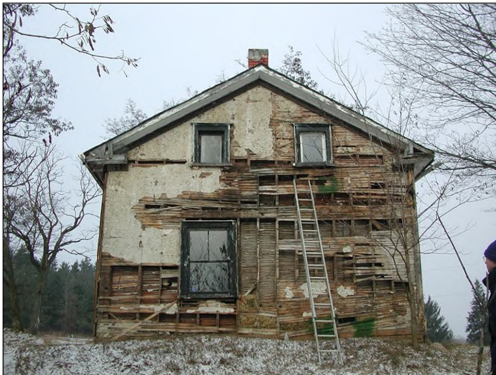
Figure 10: Above: South façade showing accordion lath beneath the plaster cladding, December 2001 (Source: Andrew Stewart)
