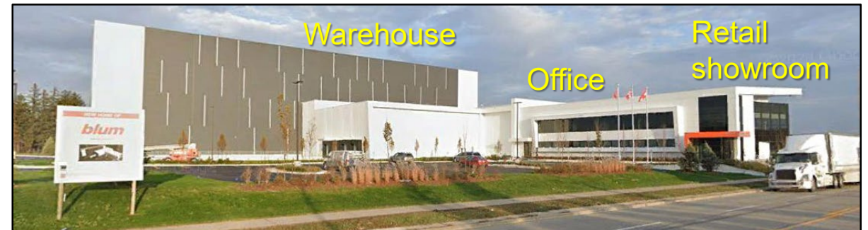
Blum Canada, Mississauga Supplier of furniture hinges, runners and lift systems. Retail showroom to demonstrate products. Office, warehouse (high ceilings, 80 ft'), retail showroom
