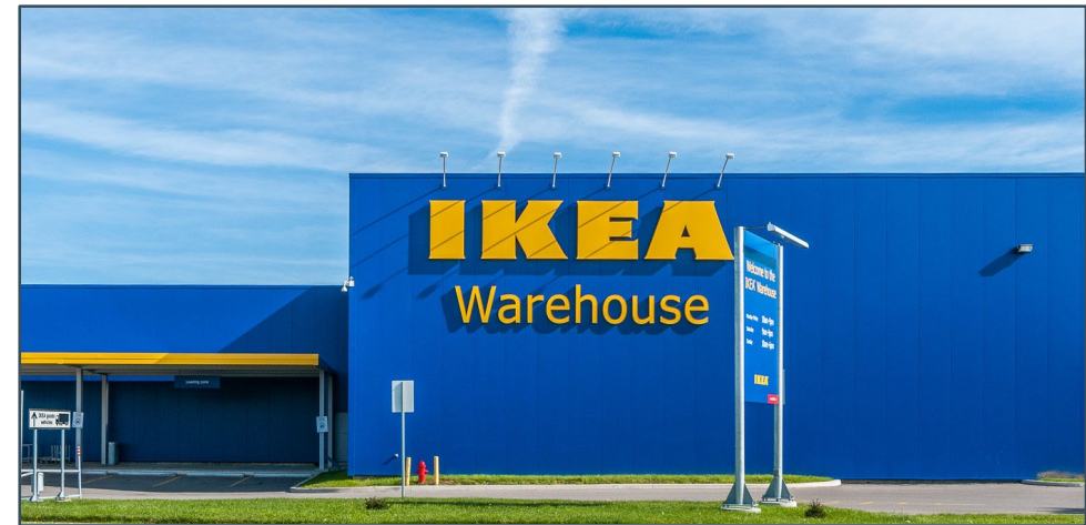
Ikea Customer Pick-up Warehouse, Toronto Reduces cost of last mile delivery.
