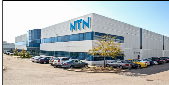
NTN Head Office and Warehouse, Mississauga
