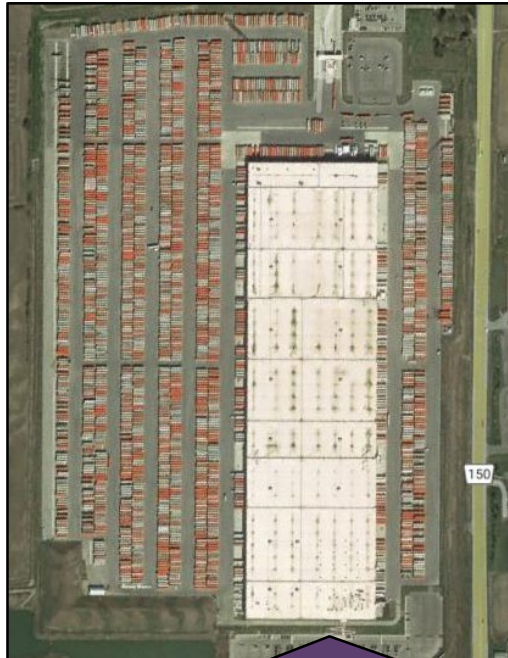
Canadian Tire Distribution Centre, Bolton, 12 jobs/ha
