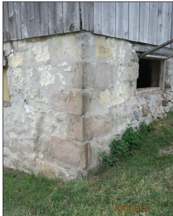
Figure 21: Below: Right: Southeast corner of barn showing red sandstone quoins and rise in grade to the north. June 2021 (Source: Town of Caledon)
