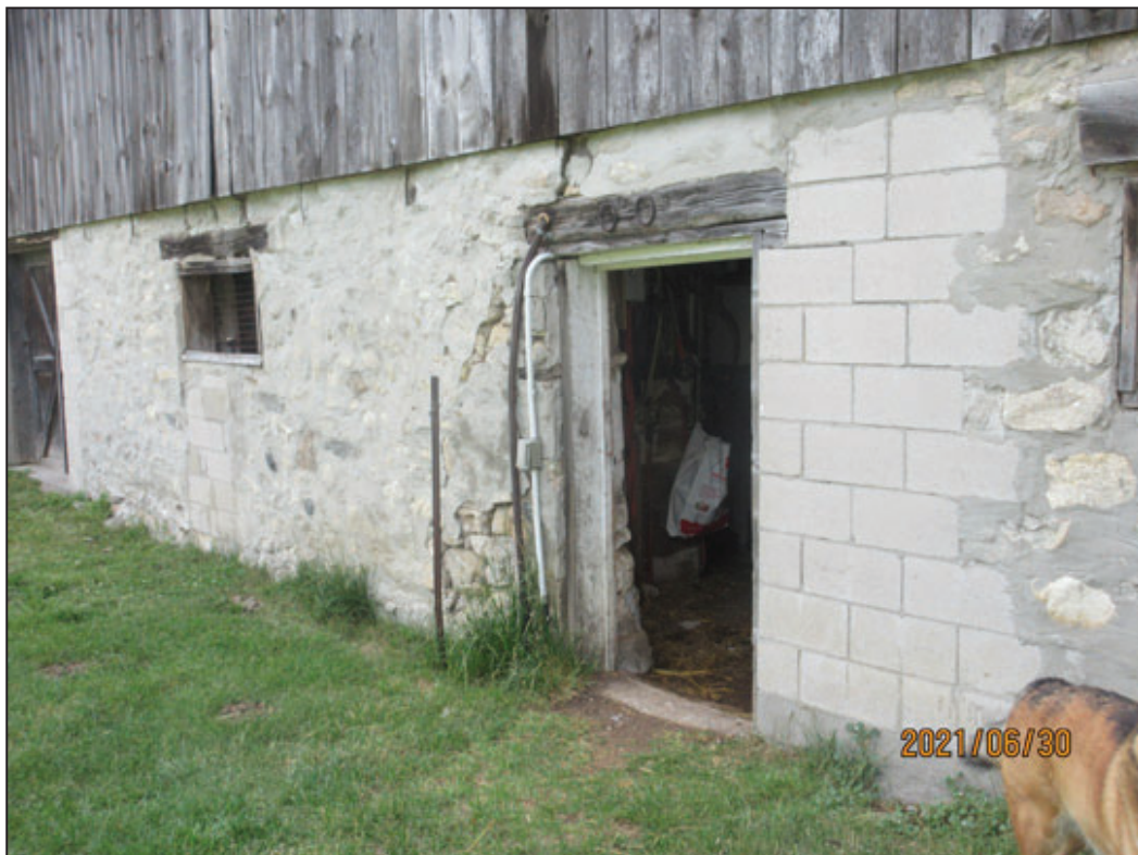
Figure 18: Below: Barn, south façade foundation showing original stone and sections of concrete block repair, June 2021 (Source: Town of Caledon)
