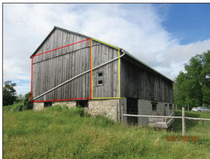
Figure 23: West façade of barn indicating the main section (red) and extension (yellow) creating the saltbox form (Source: Town of Caledon)
