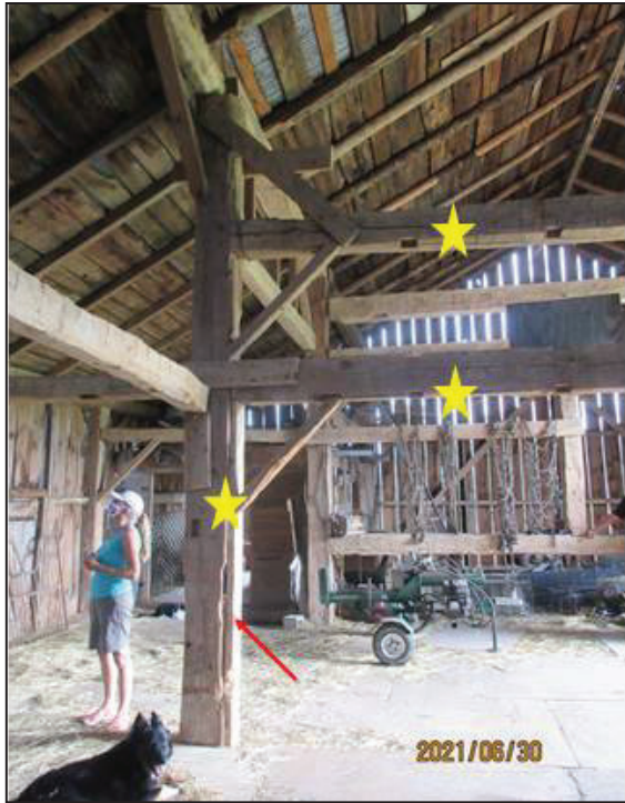
Figures 23 and 24: Barn interior with yellow stars indicating locations of some removed girt studs and corner braces. The red arrow indicates where a mortise for a removed lower girt has been covered with planks. The red circle indicates repositioning of the north end of the middle girt. (Source: Town of Caledon)
