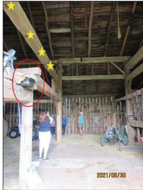
Figures 23 and 24: Barn interior with yellow stars indicating locations of some removed girt studs and corner braces. The red arrow indicates where a mortise for a removed lower girt has been covered with planks. The red circle indicates repositioning of the north end of the middle girt. (Source: Town of Caledon)
