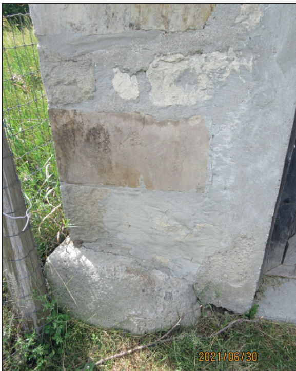
Figure 21: Below: Right: Southeast corner of barn showing red sandstone quoins and rise in grade to the north. June 2021 (Source: Town of Caledon)
