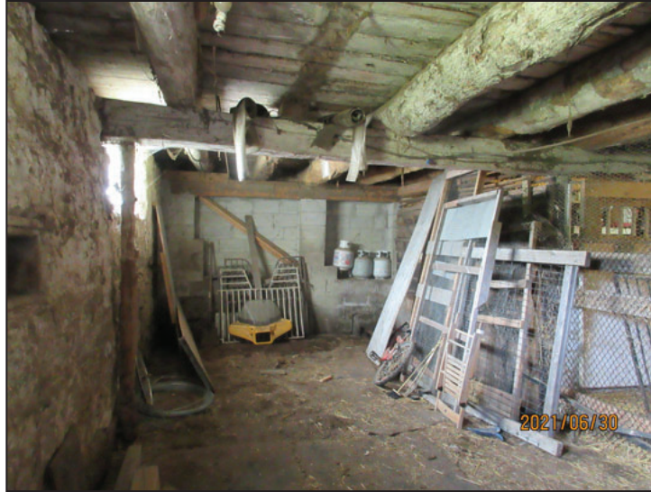
Figure 30: Above: Barn, looking north along west end stone foundation wall (left) at concrete block repairs on north foundation wall, June 2021 (Source: Town of Caledon)
