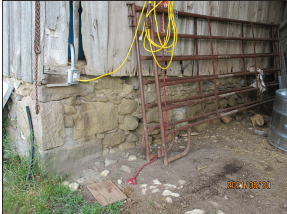
Figure 19: Above: Barn, northeast corner showing red sandstone quoins and section of original siding. Note lower height of foundation wall compared to south façade due to change in grade, June 2021 (Source: Town of Caledon)
