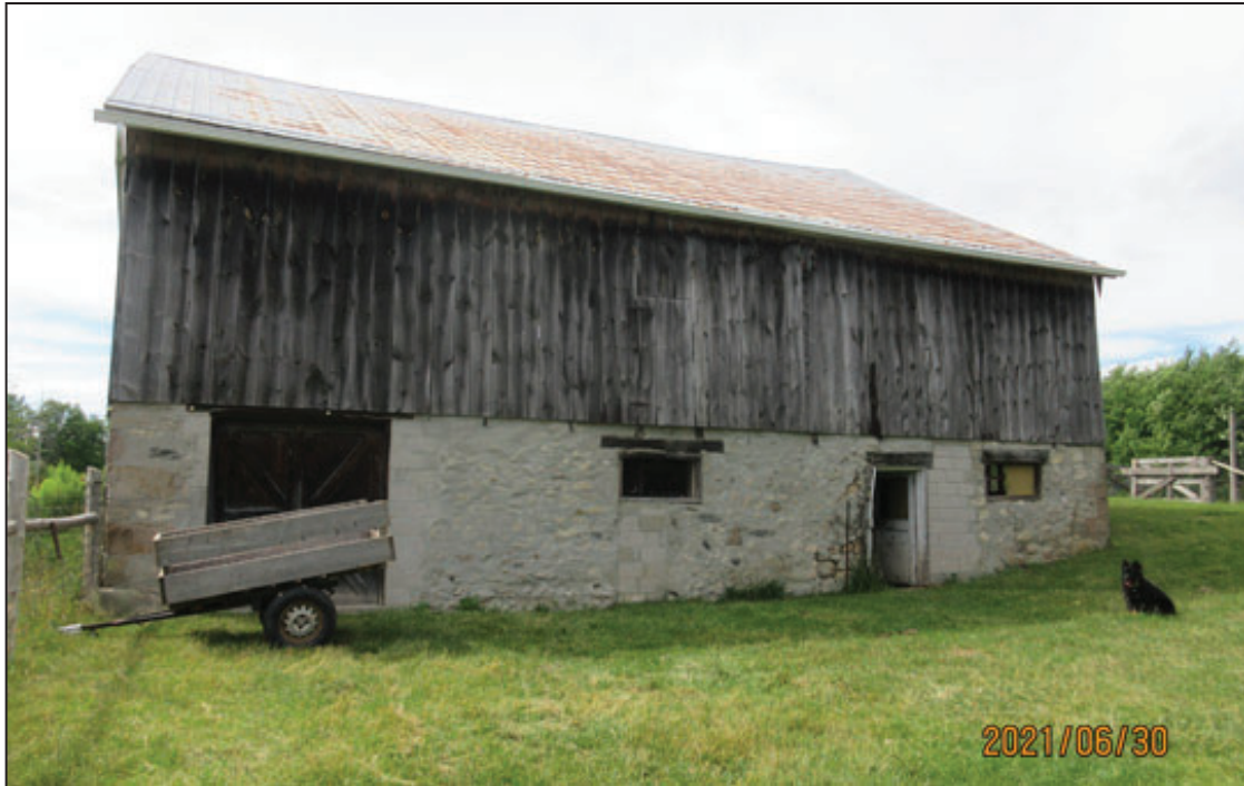
Figure 17: Above: Barn, south façade, showing stone foundation / stable area set into natural slope at east end, June 2021 (Source: Town of Caledon)
