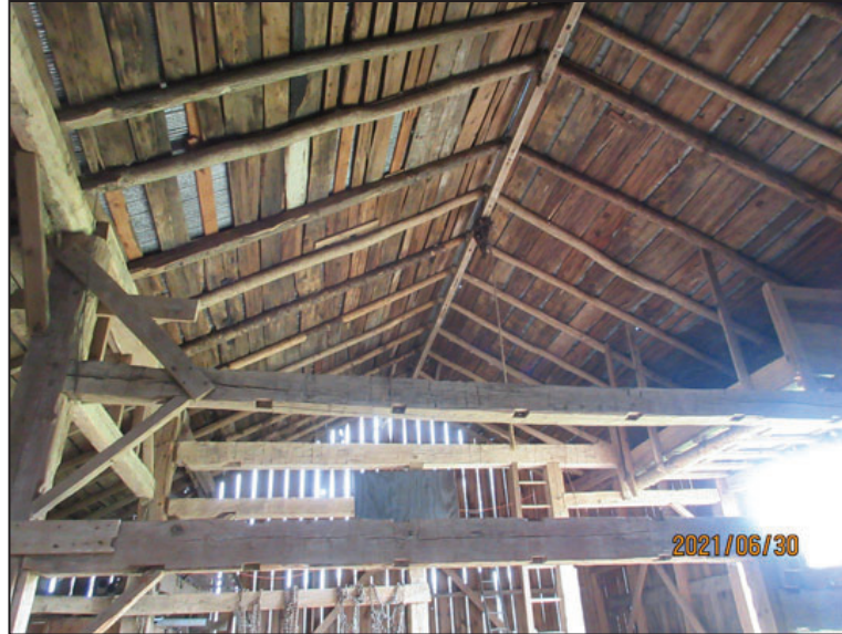
Figure 27: Above: Barn, looking west at interior bents. Note pole rafters and original roof sheathing, June 2021 (Source: Town of Caledon)
