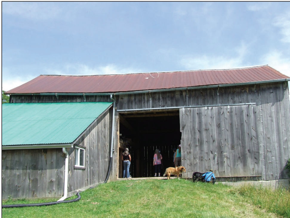
Figure 16: Below: Barn, north façade showing earth ramp and drive door accessing the centre bay threshing floor, June 2021 (Source: Town of Caledon)
