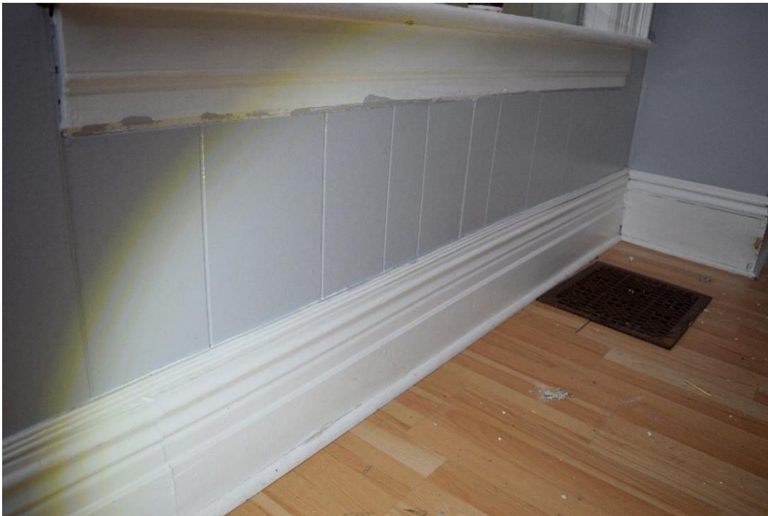
Image 48: Typical original baseboard found on first floor
