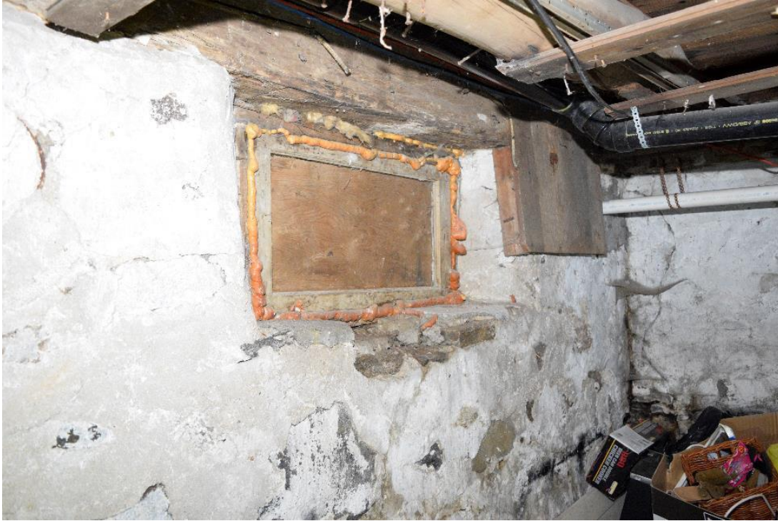
Image 41: Original window in basement, note large square timber at top of foundation wall
