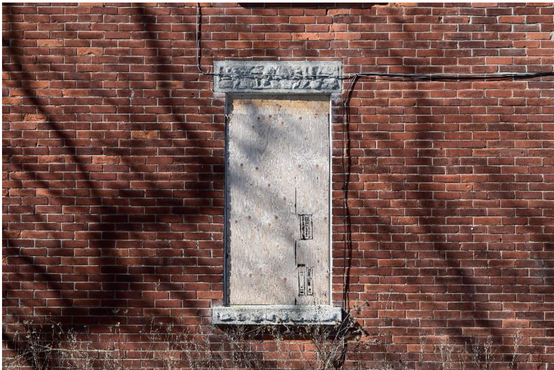
Image 14: Typical window opening in original structure, note decorative cast concrete lintel and lug sill
