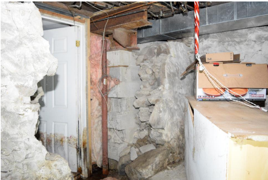
Image 40: Connection between original basement and addition, note presence of original field stone foundation and concrete masonry units used for foundation of addition
