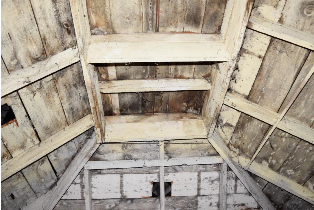
Image 45: Typical framing associated with truncated hip roof
