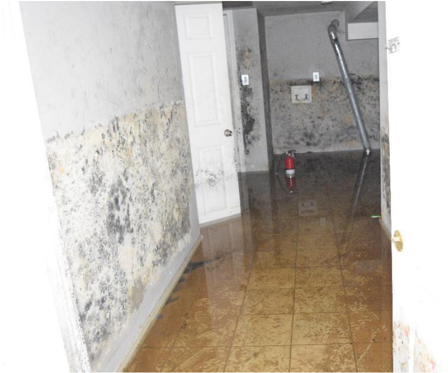
Image 43: Flooding in basement of rear addition
