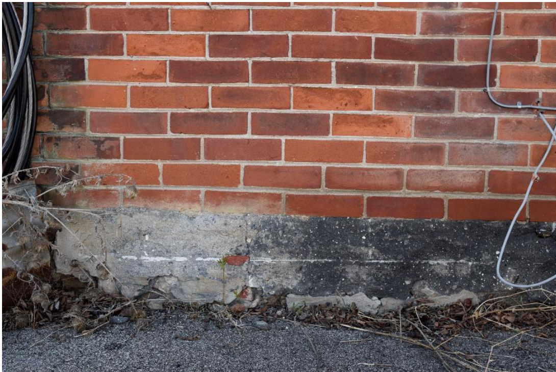
Image 22: Typical wall finish, smooth red brick with tooled mortar joints atop rubble stone foundation with concrete finish tooled to resemble cut stone
