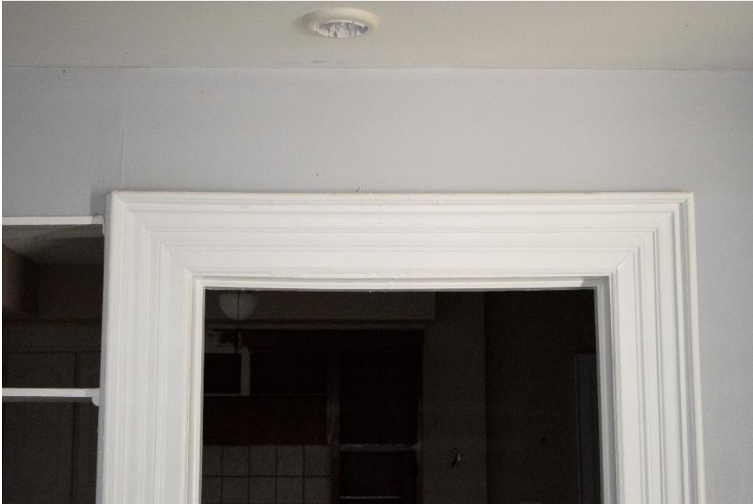
Image 47: Example of original door trim as found on first floor
