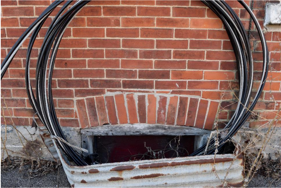
Image 15: Segmentally headed window in foundation of original structure
