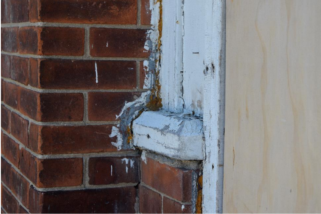
Image 19: Connection between closed porch and main house, mortar joints align indicating congruent construction, and that porch is original to the structure
