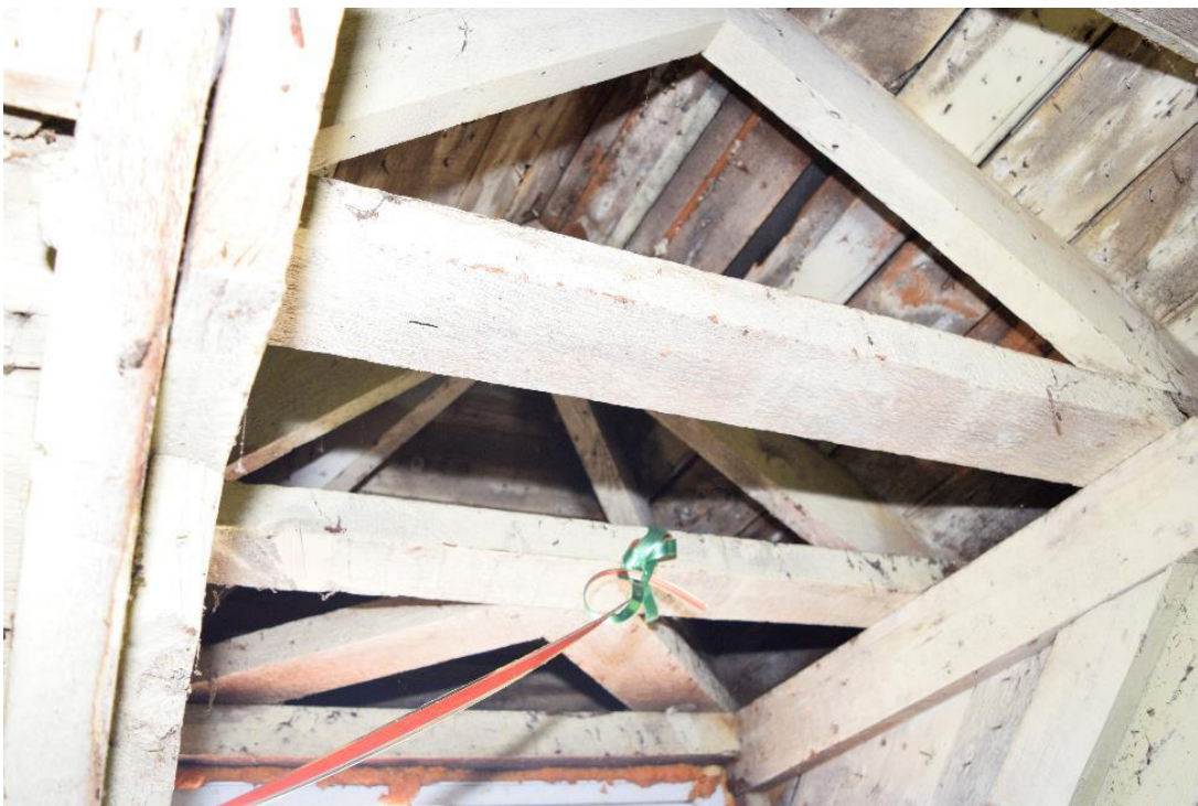
Image 46: Framing of rear hip gable
