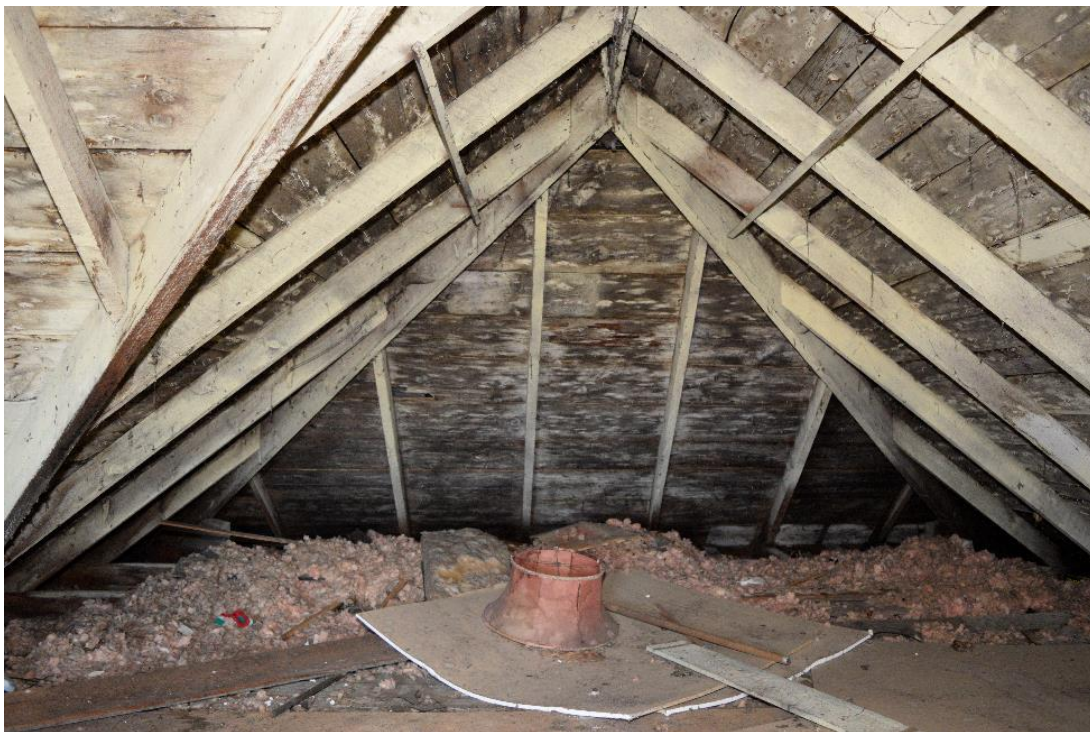
Image 44: Typical roof framing
