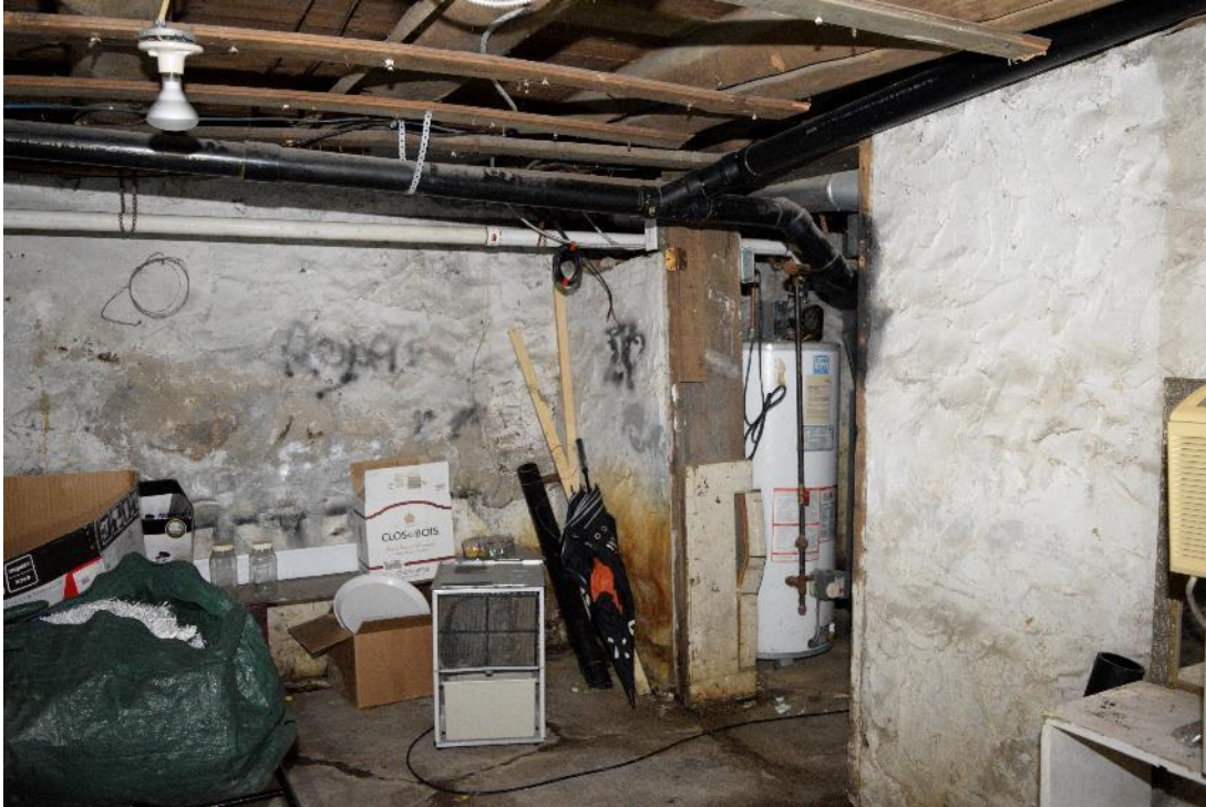
Image 39: Field stone foundation with lime wash, typical of basement, facing north
