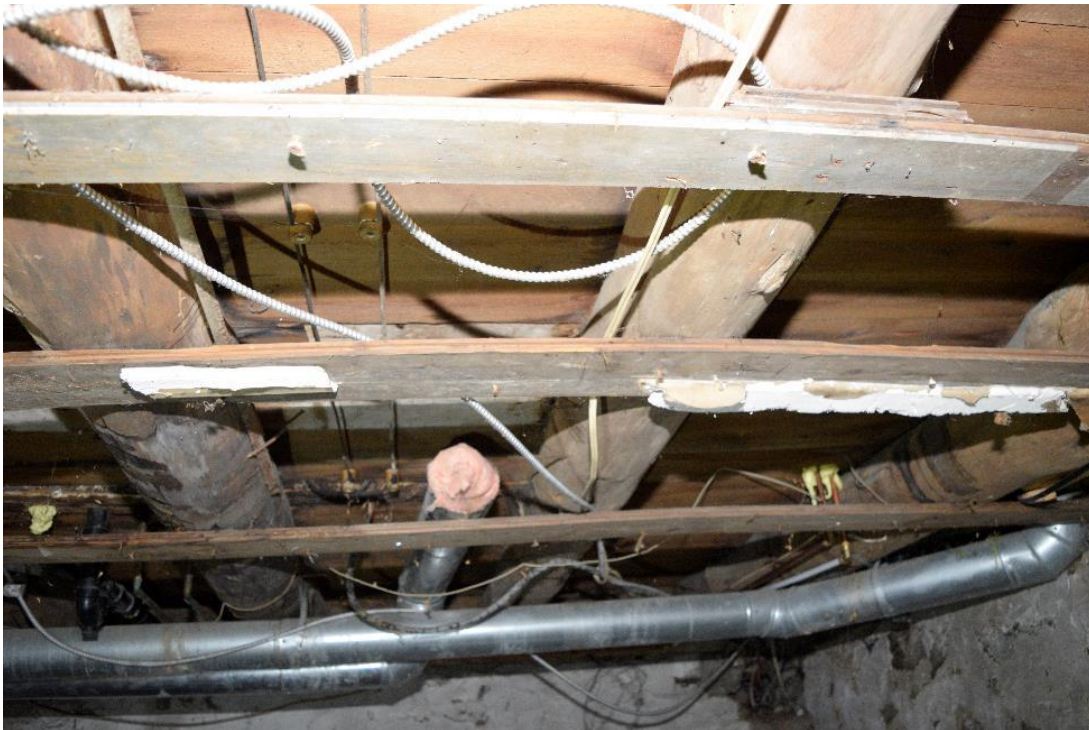
Image 42: Typical floor construction, joists are full round logs with tongue and groove floorboards
