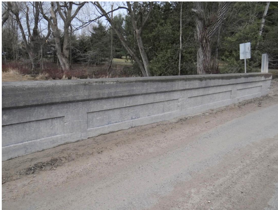
Plate 18: East parapet wall, handrail, and decorative panelling of the Kennedy Road Bridge, looking southeast
