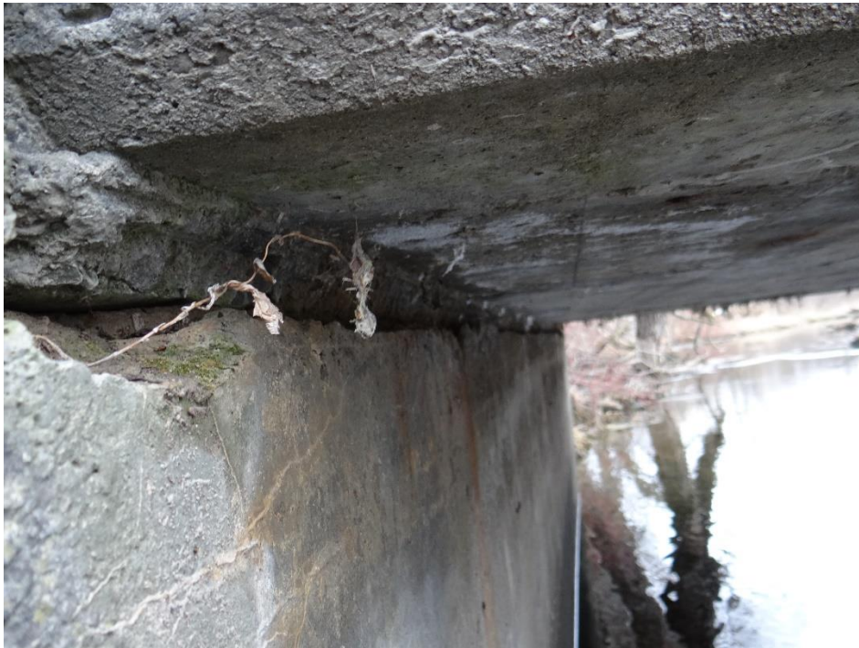
Plate 14: View of south abutment expansion gap from the southeast corner, looking west
