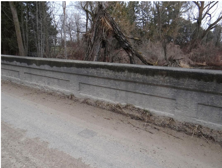
Plate 20: West parapet wall, handrail, and decorative panelling of the Kennedy Road Bridge, looking southwest
