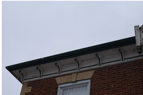
Plate 10: Details of decorative wood brackets and wood fascia, looking east
