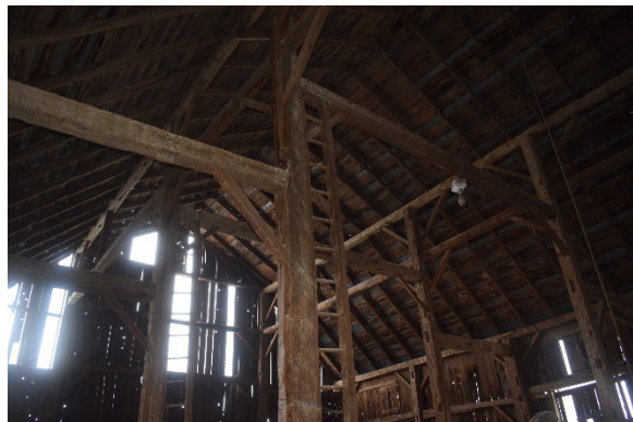
Plate 38: Interior of loft area showing hand hewn beams, posts, and joints, looking east
