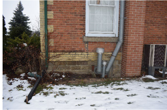
Plate 17: Buff brick quoins, buff brick band, cut coursed ashlar stone foundation, and utility conduits, looking north
