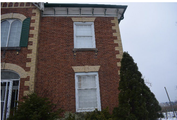
Plate 11: Modern 8/8 windows and 8/12 windows, with buff brick voussoirs and stone sills, looking east
