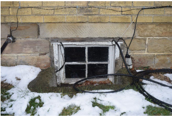
Plate 22: Four pane wood frame basement window, looking south
