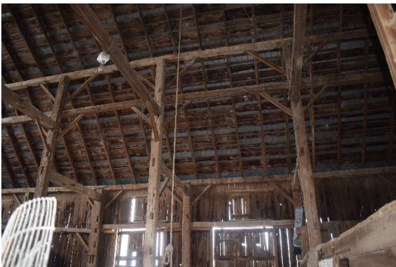
Plate 37: Interior of loft area showing hand hewn beams, posts, and joints, looking south
