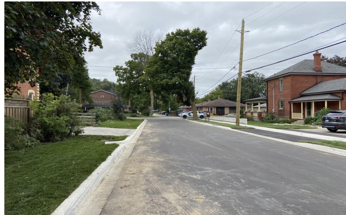
Albert Street After Reconstruction
