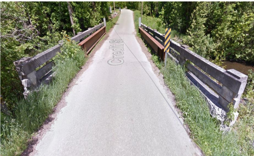
Credit St Bridge Before Replacement
