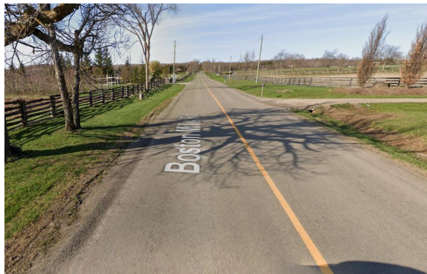
Surface Treatment (Boston Mills Rd)
