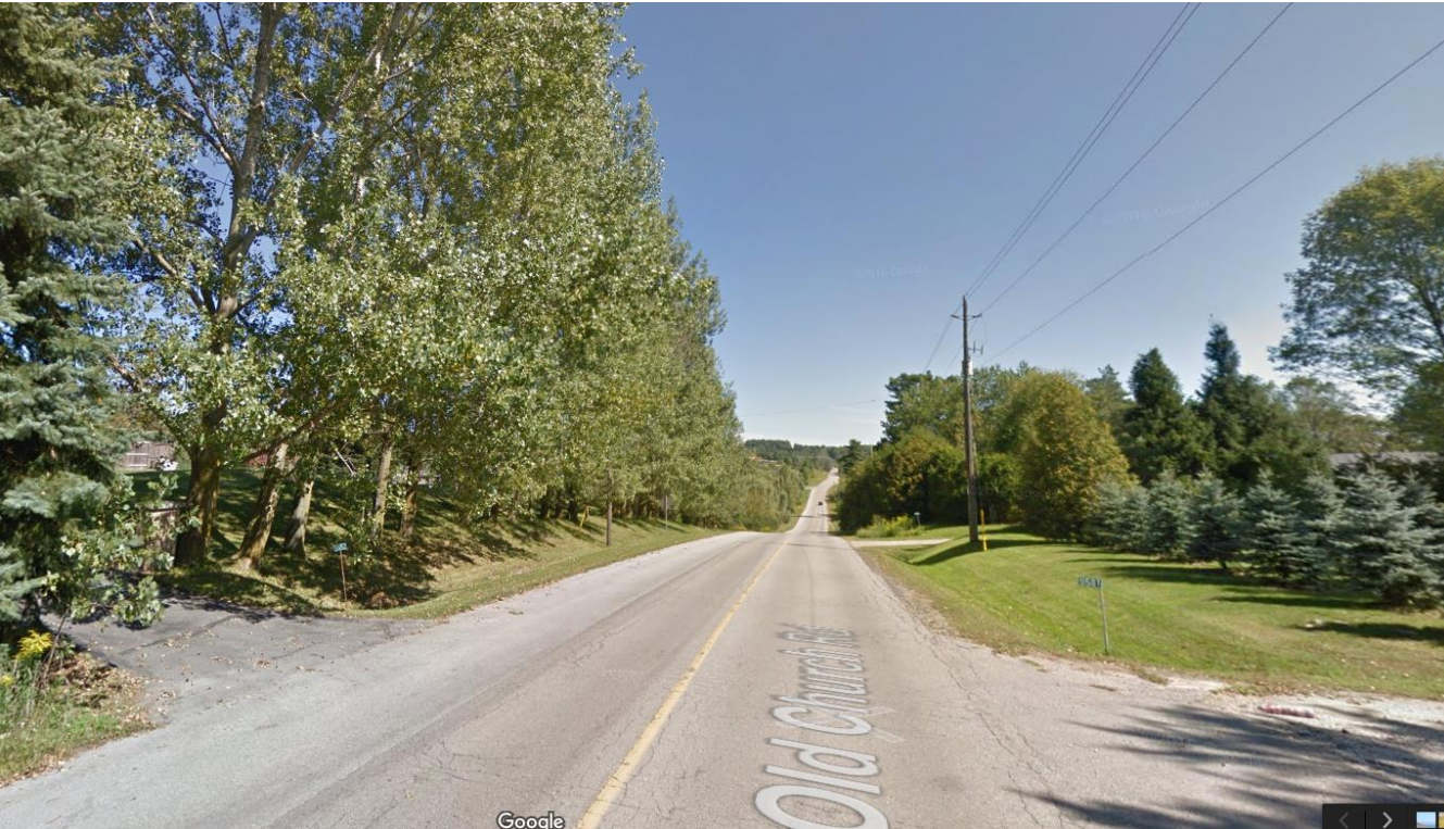
Old Church Rd Before Reconstruction
