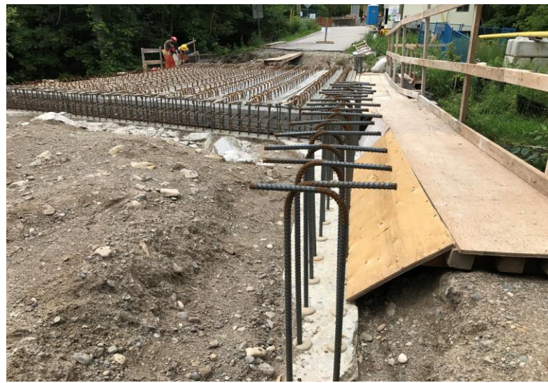
Credit St Bridge During Replacement
