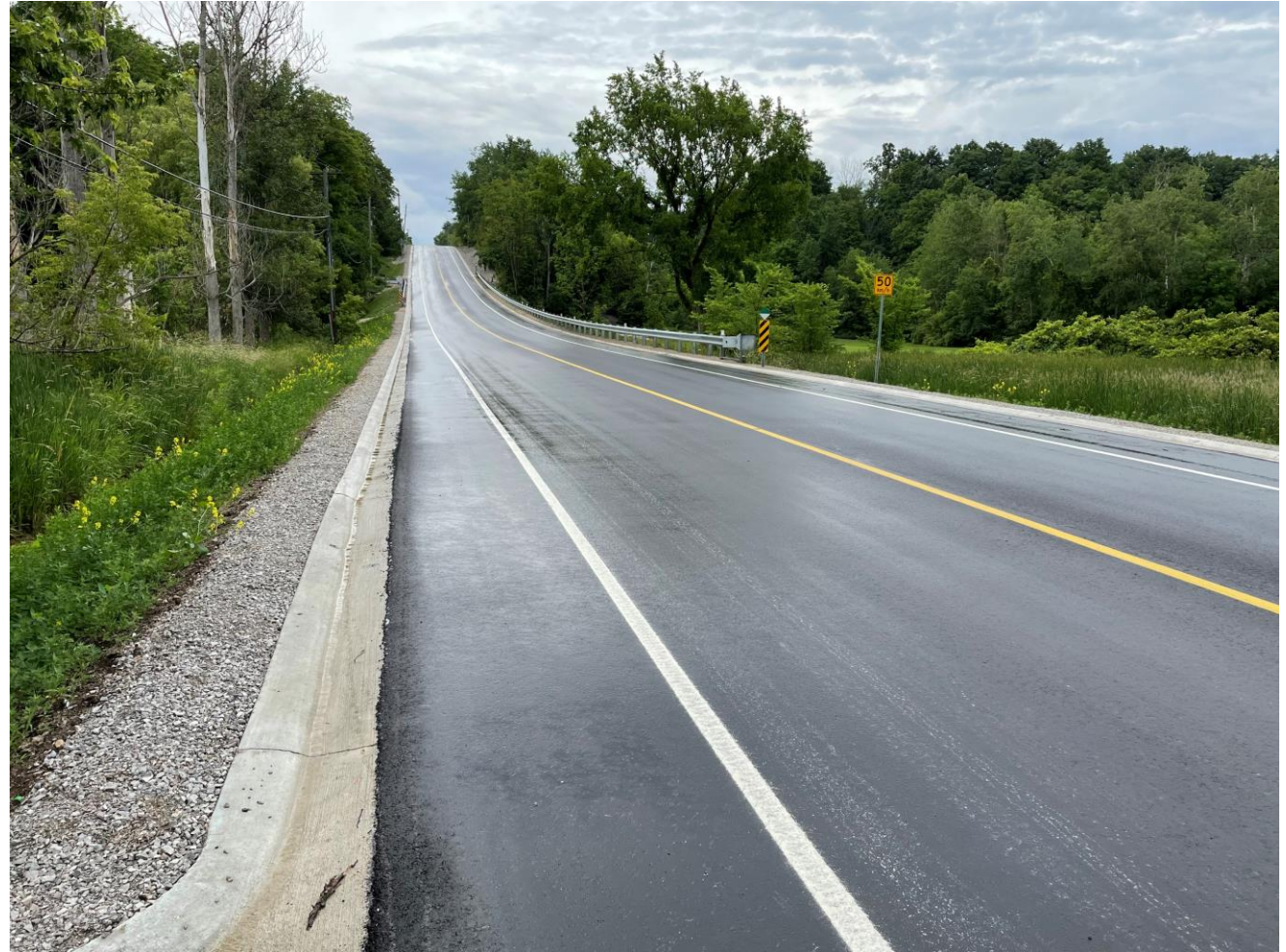
McLaughlin Road post reconstruction
