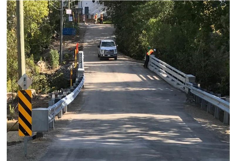
Credit St Bridge After Replacement
