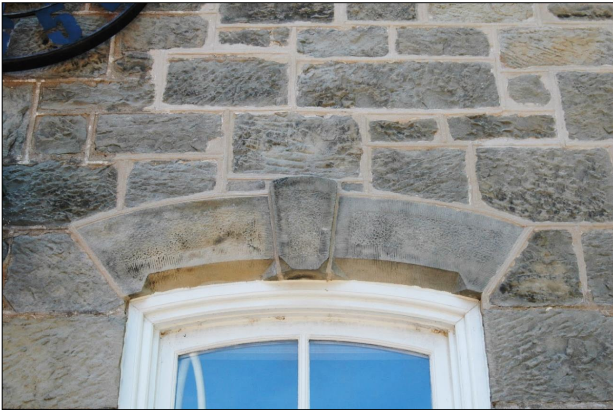
Image 7: Sharpe Schoolhouse: repointed areas of exterior stonework
