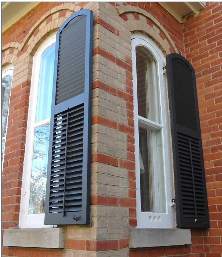
Image 4: Little-Webber House: repaired and repainted shutters
