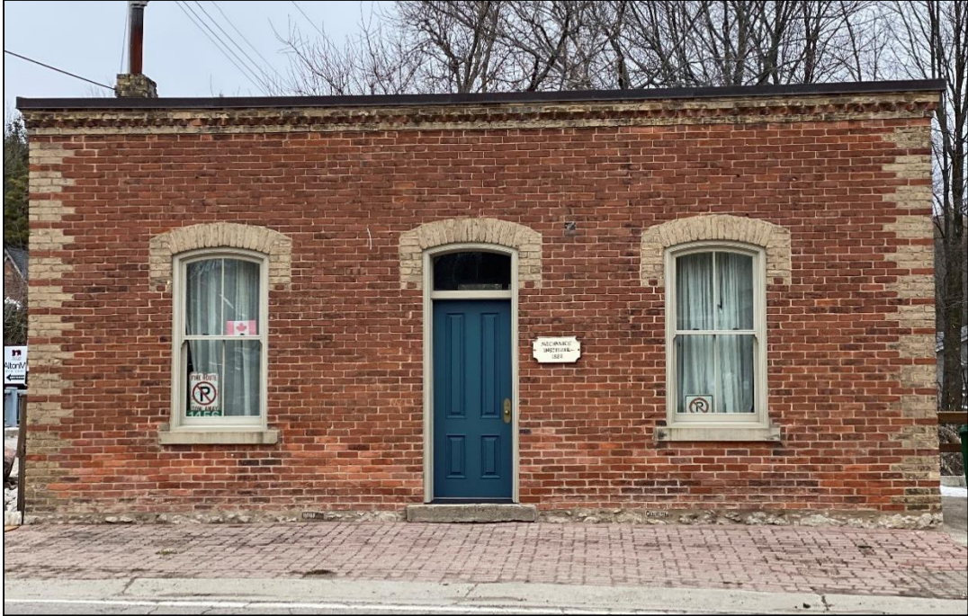
Image 1: Alton Mechanics Institute: repaired roof and flashing; repointed brickwork; replaced windows and front door
