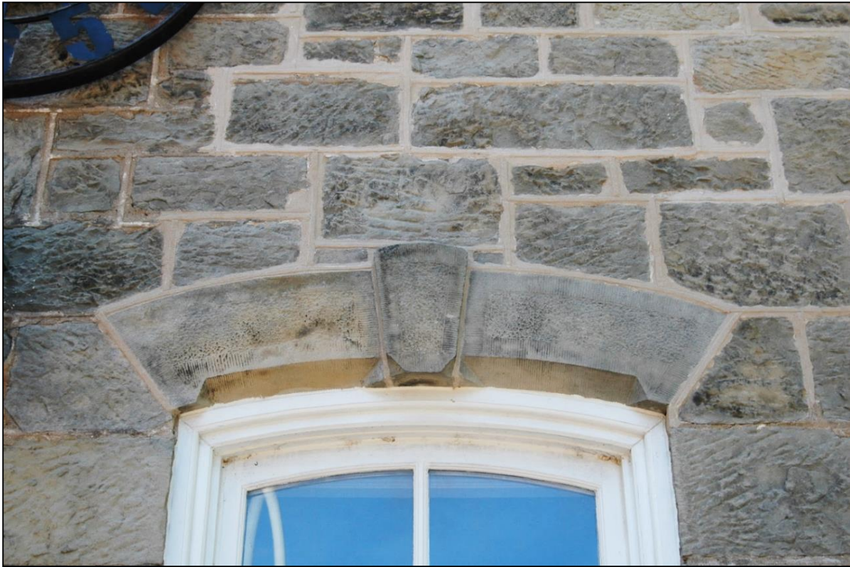
Image 7: Sharpe Schoolhouse: repointed areas of exterior stonework
