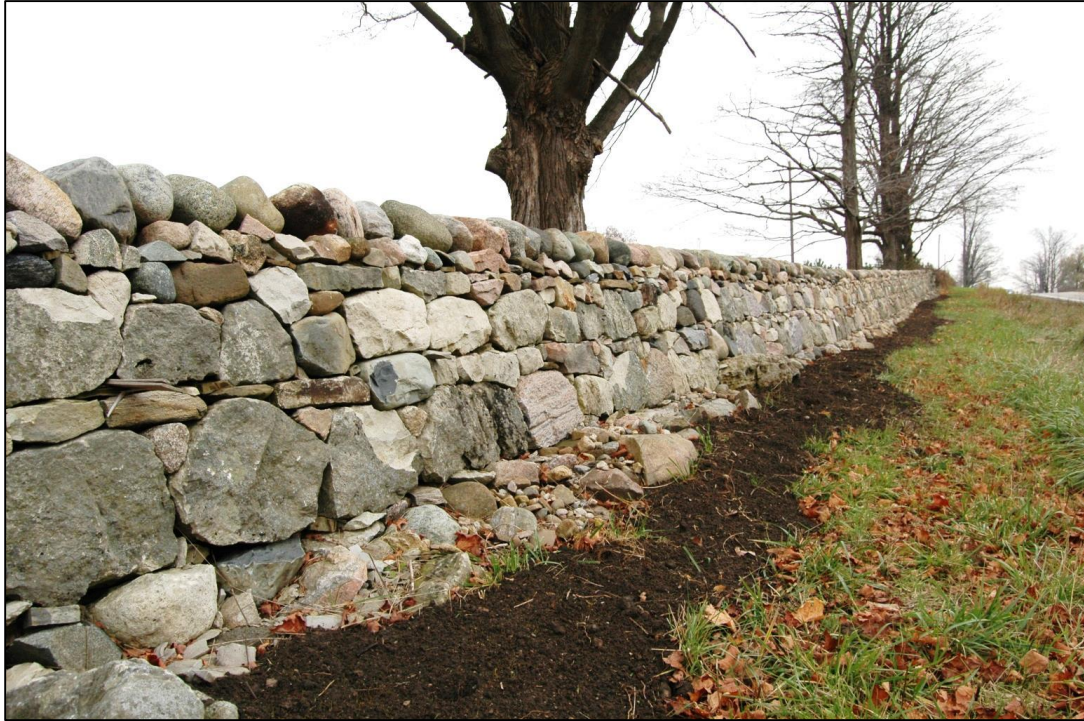
Image 11: Patullo-McDiarmid Dry Stone Wall: restored using existing stone and new cedar shakes.
