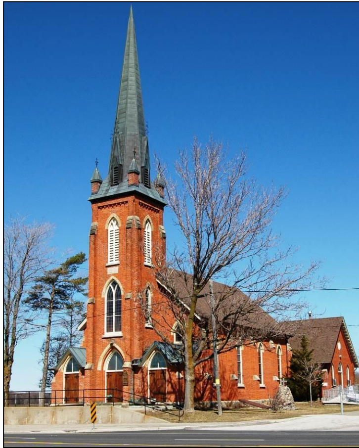
Image 9: Claude Presbyterian Church: repaired front gable fascia and soffits; painted exterior wood trim and exposed rafters in eaves
