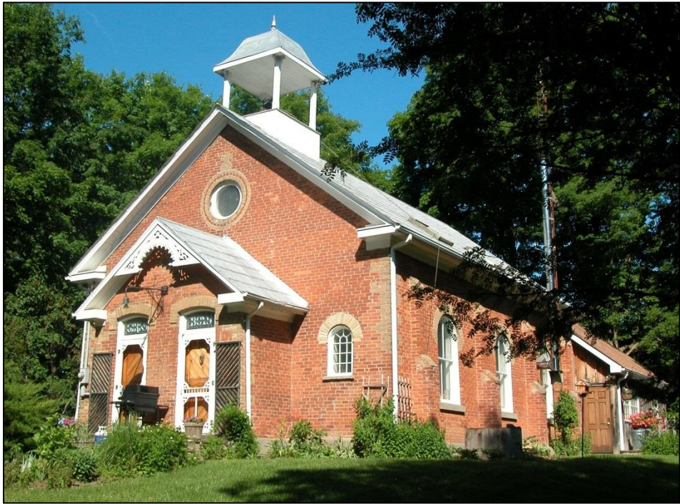
Image 10: Silver Creek Schoolhouse: repaired fascia, soffits, and bell tower
