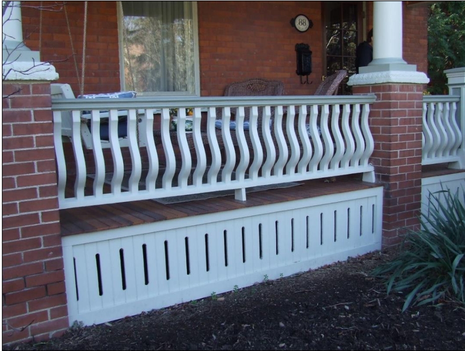
Image 3: Bolton Heritage Conservation District: restored front porch elements
