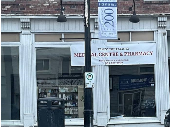
56 Queen St N, Bolton Approved for: Sign (Note: Owner replacing top board of façade this spring)
