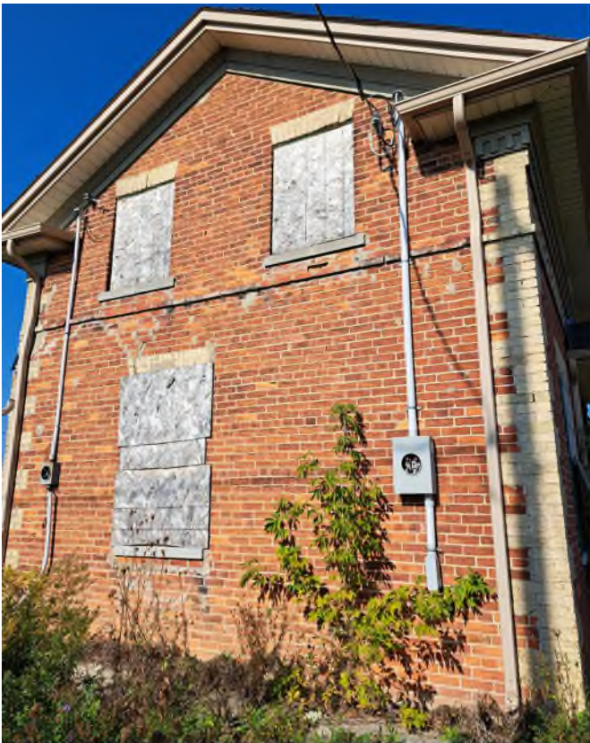
Figure 8: Side (south) façade of the Thompson-Scott House, October 2023
