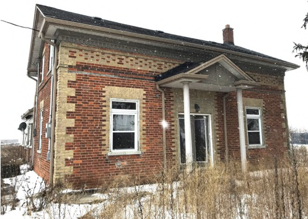
Figure 6: Front (east) façade of the Thompson-Scott House, January 2019.
