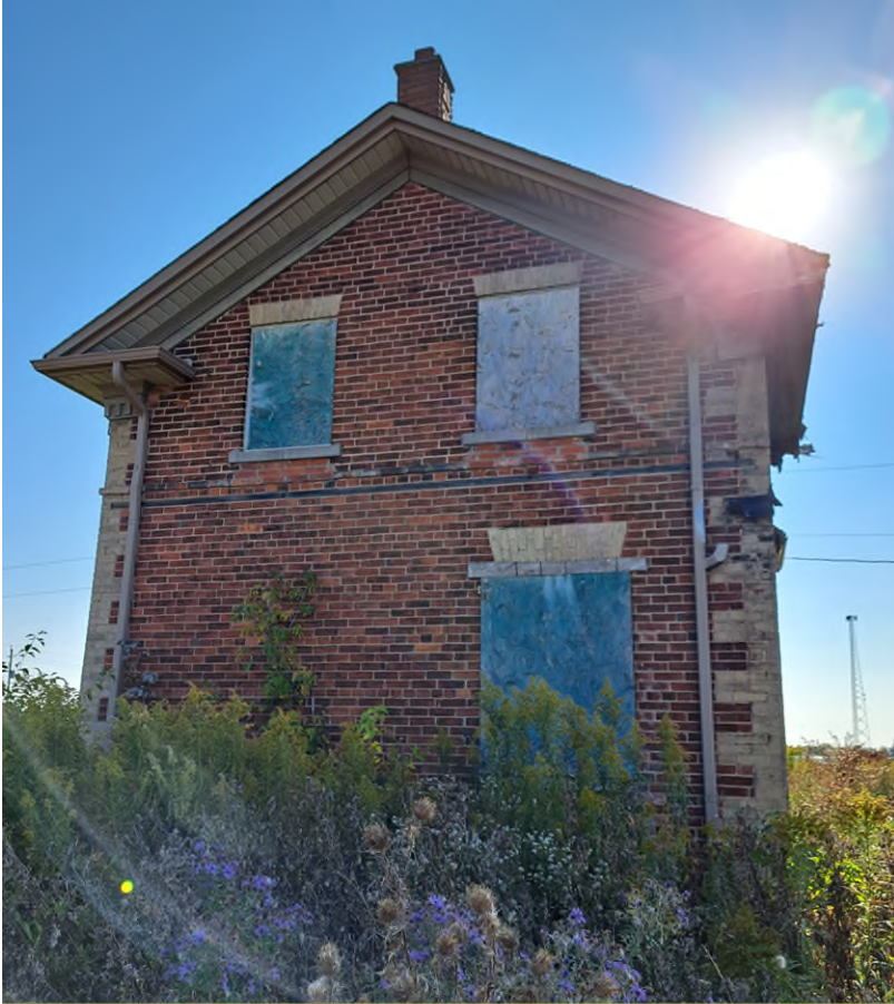
Figure 9: Side (north) façade of the Thompson-Scott House, October 2023.
