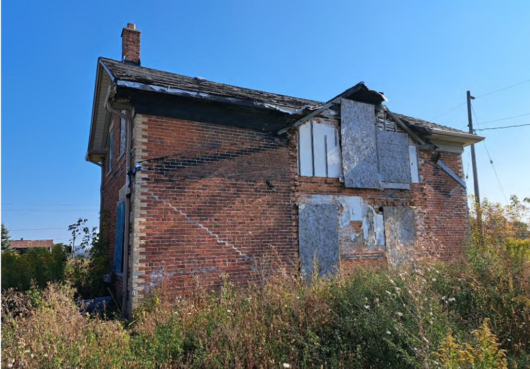
Figure 7: Rear (west) façade of the Thompson-Scott House, October 2023.
