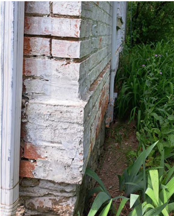
Figure 12: Details of the southeast corner of the Robinson Farmhouse, showing the narrow foundation stone and overhang of the projecting brick water table, June 2023.
