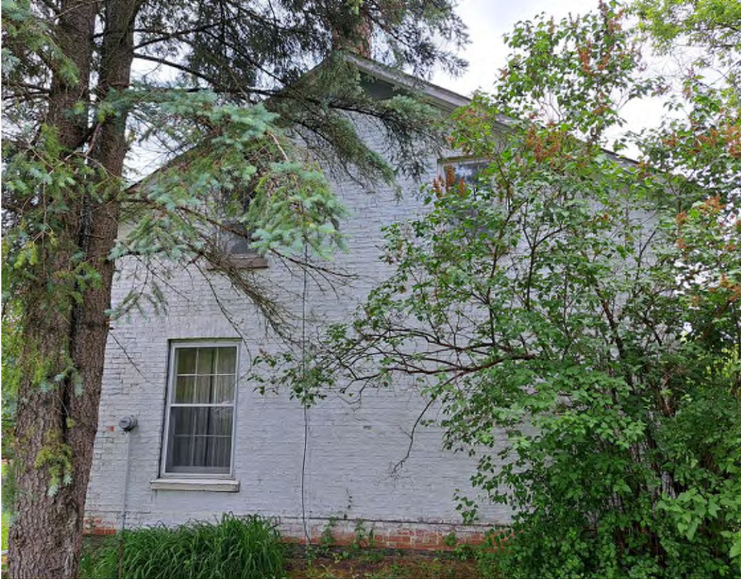
Figure 9: East (side) façade of the Robinson Farmhouse, June 2023.
