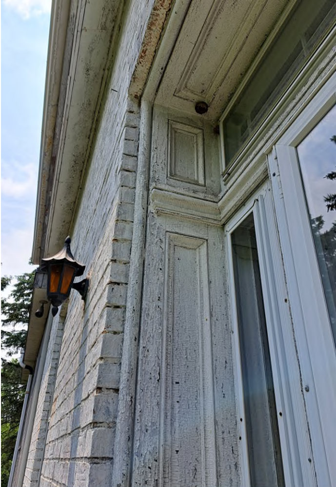
Figure 15: Detail of molded wood paneling around inset of centered entrance, June 2023.
