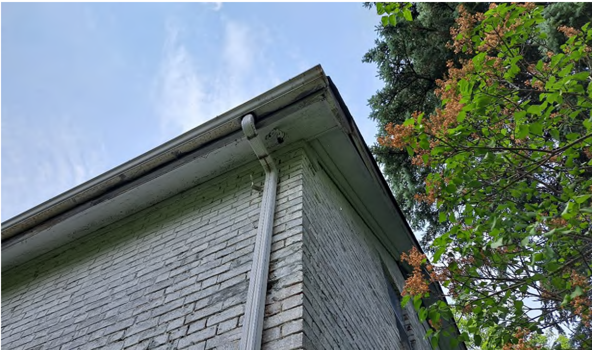
Figure 18: Detail showing wood soffits and moulded fascia in gable ends, June 2023.
