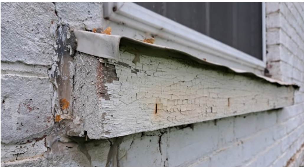
Figure 16: Wood lug sill beneath extant double hung wood sash window, June 2023.
