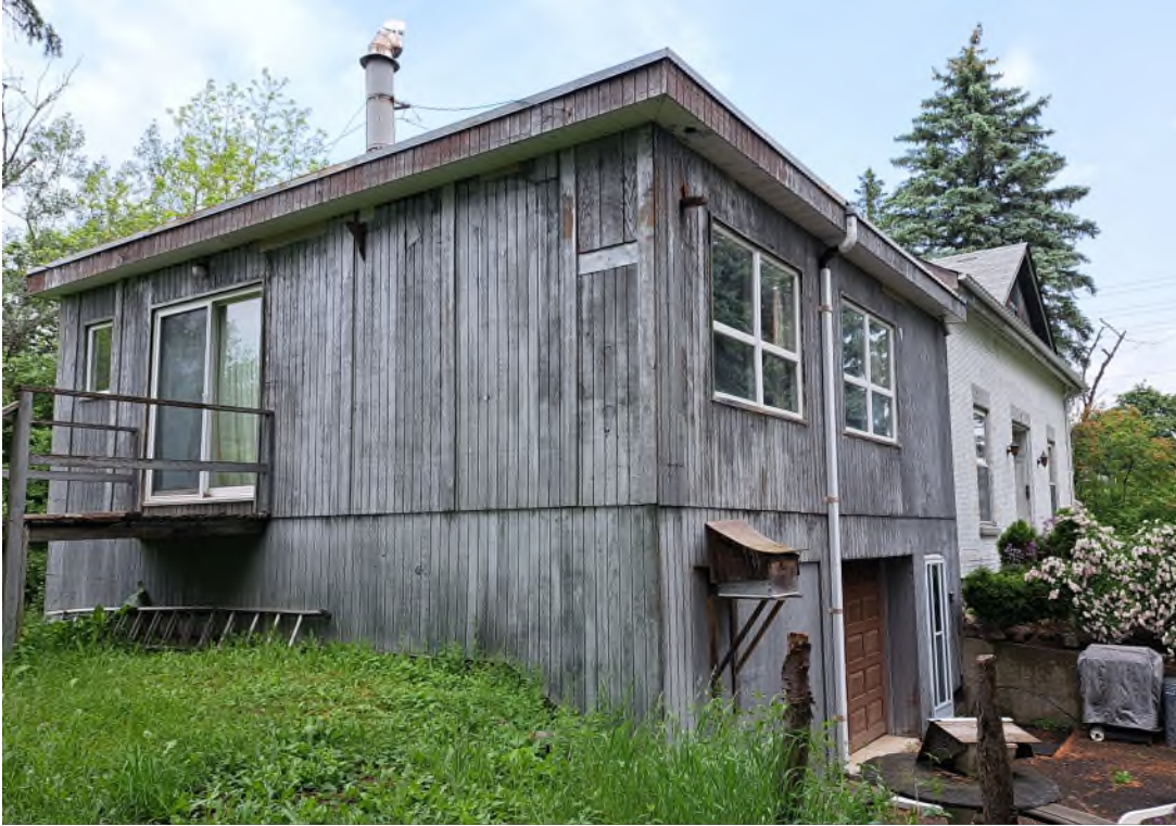
Figure 11: West and south façades of the Robinson Farmhouse, showing the modern addition, June 2023.
