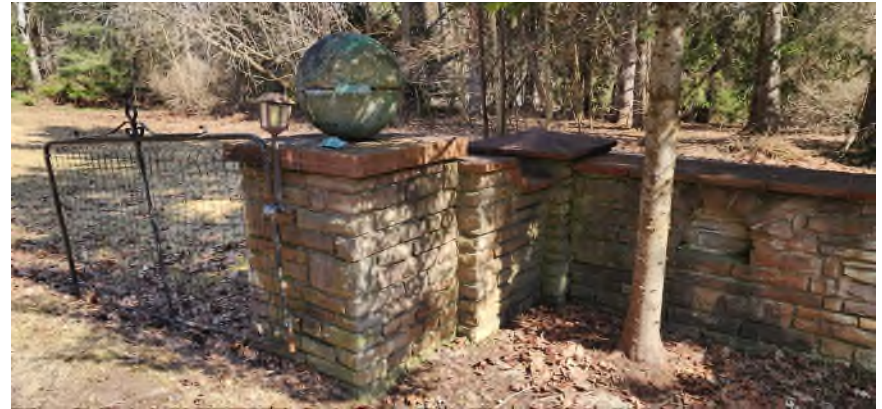
Figure 36 - Right gate post. (Photo: RHC 2024)
