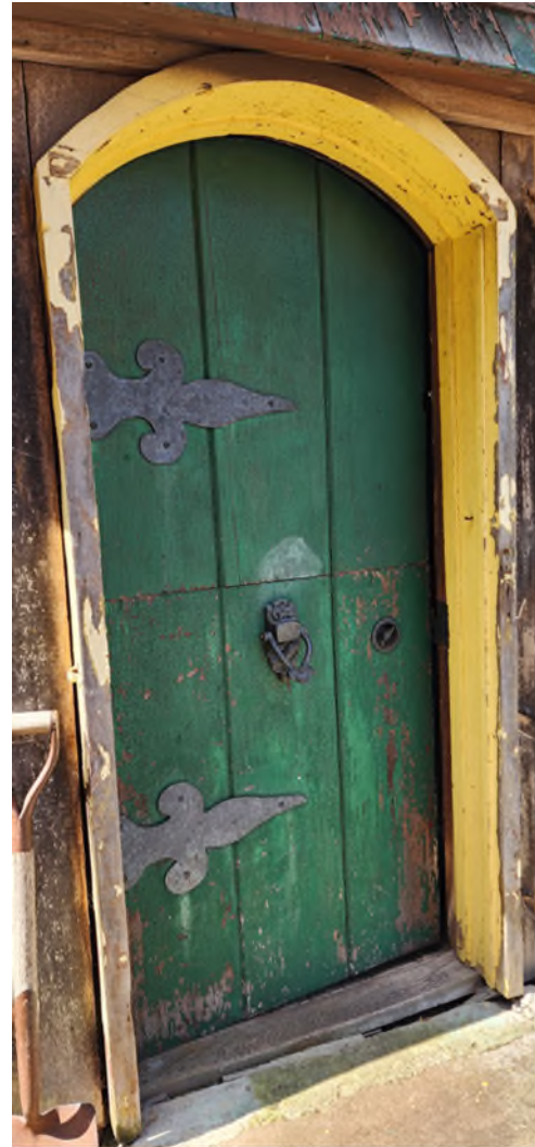
Figure 20 - Front door. (Photo: RHC 2024)
