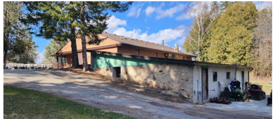
Figure 47 - Barn foundation beside modern golf clubhouse. (Photo: RHC 2024)
