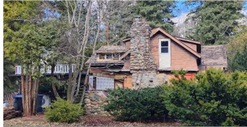
Figure 22 - West elevation from driveway. (Photo: RHC 2024)
