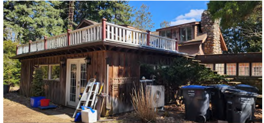
Figure 27 - North elevation with stairs to addition roof. (Photo: RHC 2024)
