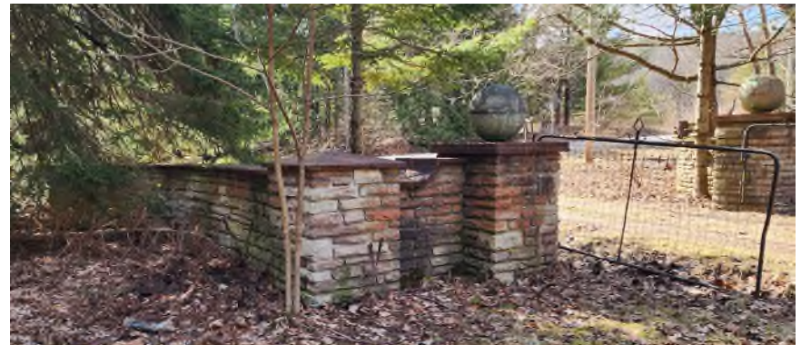
Figure 37 - Rear of right gate wall. (Photo: RHC 2024)
