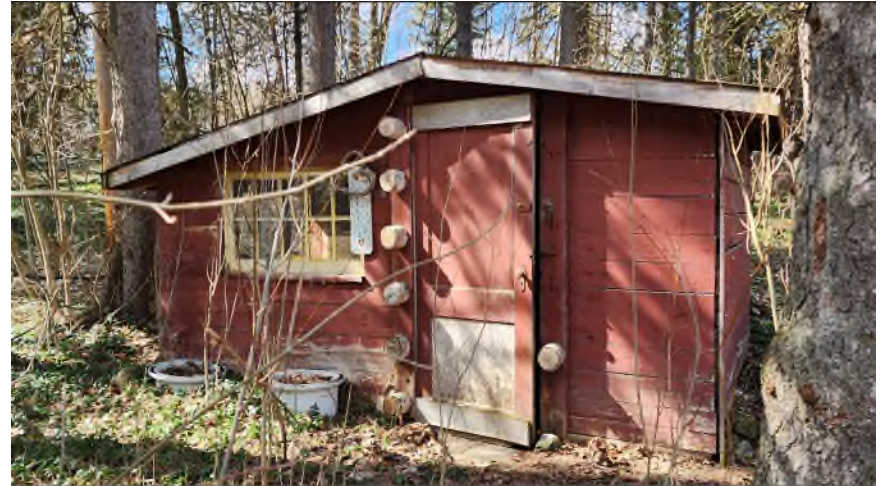
Figure 46 – Shed from driveway. (Photo: RHC 2024)
