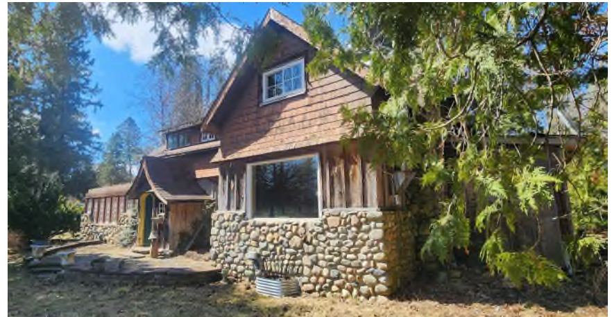
Figure 15 - Front gable from east. (Photo: RHC 2024)
