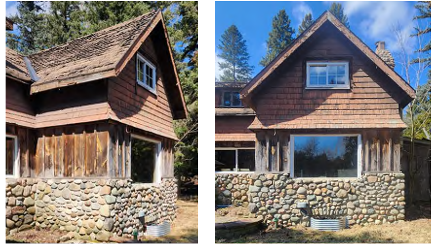
Figure 21 - Front gable. (Photo: RHC 2024)
