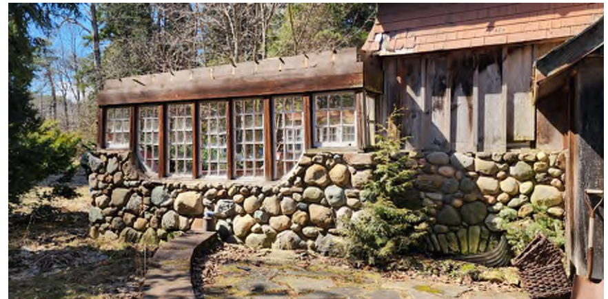
Figure 17 - Front of conservatory. (Photo: RHC 2024)
