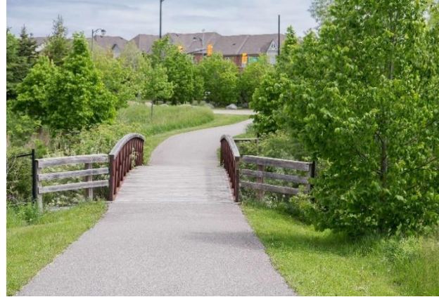
Example of a multi-use trail outside of the road right-of-way (Caledon, ON)
