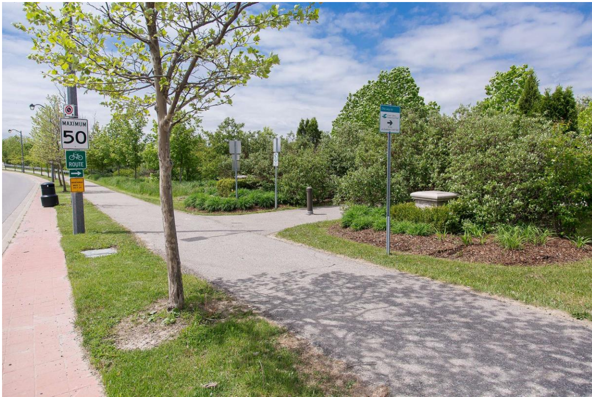
Picture 19. Multi-use path on Kennedy Road
