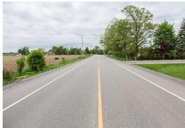
Example of a paved shoulder (Caledon, ON)
