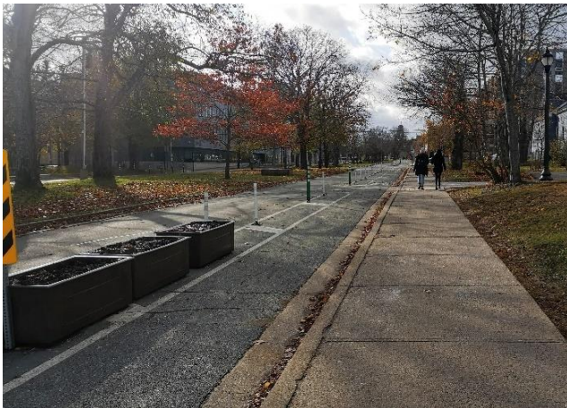
On-road protected bikeway with planters and flex posts (Halifax, NS)
