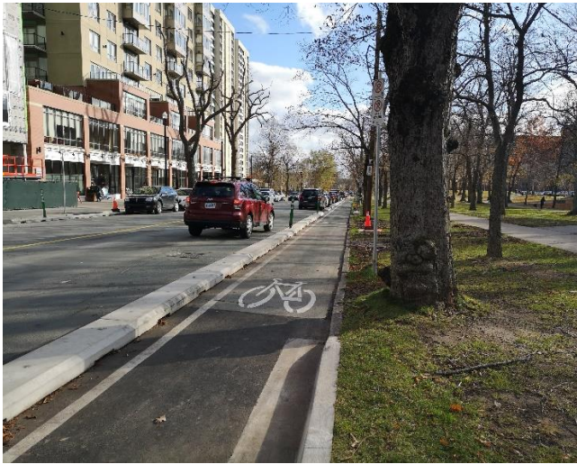
On-road protected bikeway with concrete curb (Halifax, NS)
