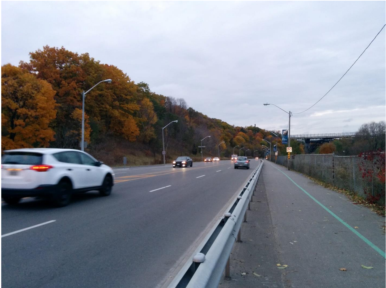
At-grade multi-use path separated with guardrail (Toronto, ON)
