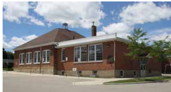
South-east corner with views of east and south elevations(ERA 2018).
