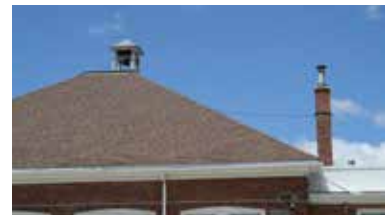
Roof, bell tower and chimney (ERA, 2018).
