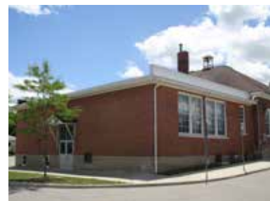
Flat roof of the 1908 building addition (ERA, 2018).
