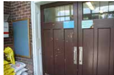
Original front doors (ERA, 2018).
