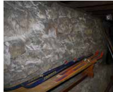
Stone Foundation as seen from the basement(ERA, 2018).
