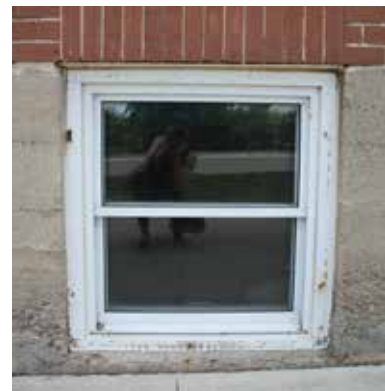
Basement window on north wall (ERA, 2018).
