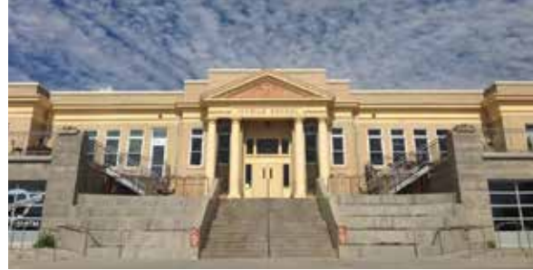
Ivywild School - Exterior ( https://stayoutwest.com/2018/02/the-principals-office/ )
