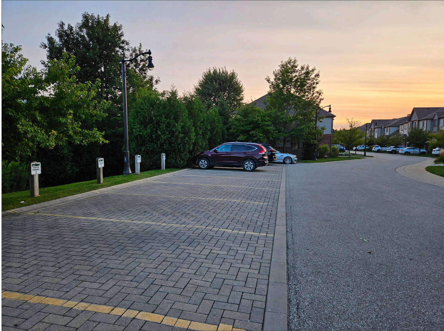
Permeable Paver Parking, Downey Trail - Seaton Group
