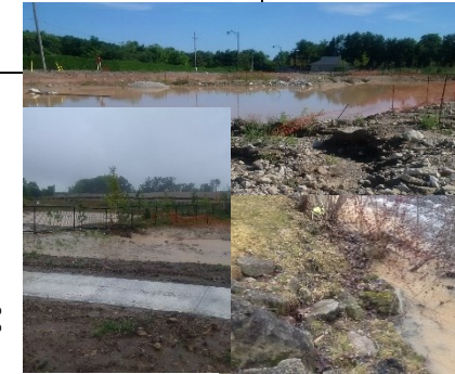
2016 Alton: Rain intensity exceeding 100 year storm intensity resulting in an unassumed pond failure and sediment discharge
